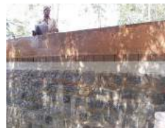
STONE FOUNDATION WITH MUD BRICKS, RAMMED EARTH WALLS CAN HOLD WELL IN PLACE ON ITS OWN WEIGHT, THE MUD BRICKS ARE THERE FOR DECORATION AND ARE OPTIONAL.
