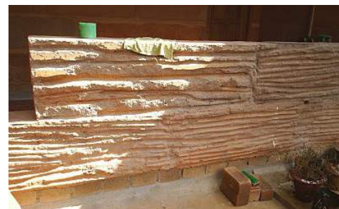
EARTH CAN BE RAMMED INTO A LOG TYPE PATTERN, NATURAL SHADE OF COLOR IS PRESENT IN THIS IMAGE
