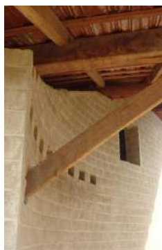
DETAILED IMAGE OF THE ROOF (SHOWS CORRUGATED DECKING, WOODEN FRAME, AND CSEB WALL WITH GAPS FOR AIR VENTILATION AND LIGHT PENETRATION).
