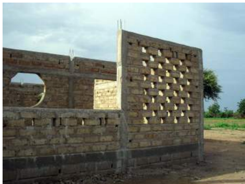
EARTH BRICK WALL IN CONSTRUCTION WITH GAPS.
