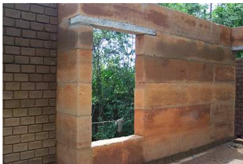
RAMMED EARTH ATTACHED TO A MUDBRICK WALL, GRANITE LINTEL IS USED ABOVE AN OPENING
