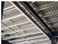
ROOF SUBSTRUCTURE BEAMS AND PURLINS
