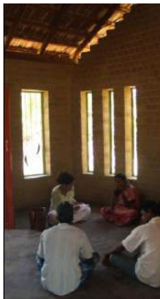
DETAILED IMAGE OF THE ROOF (SHOWS CORRUGATED DECKING, WOODEN FRAME, AND CSEB WALL WITH GAPS FOR AIR VENTILATION AND LIGHT PENETRATION).
