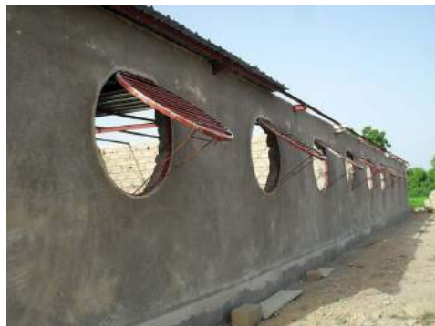
ABOVE, MOVING CLOCKWISE: SLATTED WINDOWS THAT CAN BE CLOSED OR PROPPED TO ALLOW FOR MORE LIGHT AND AIR CIRCULATION. FRONT FACADE WITH EARTH BRICKS AND CIRCULAR VOIDS FOR THE WINDOWS. SEMI ENCLOSED AREA WITH A BENCH FOR PLAY WHEN ITS TOO HOT IN THE SUN.
