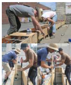
FORMWORK CONSTRUCTION
