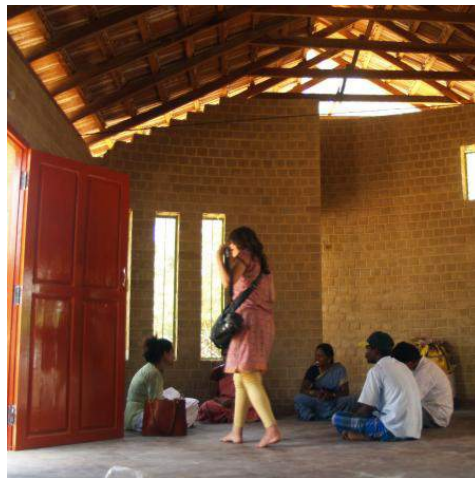
DETAILED IMAGE OF THE ROOF (SHOWS CORRUGATED DECKING, WOODEN FRAME, AND CSEB WALL WITH GAPS FOR AIR VENTILATION AND LIGHT PENETRATION).
