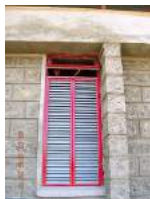
WINDOWS WITH VERTICAL SHADING DEVICES (PROTRUDING STONE UNITS), SHUTTERS, AND AN UPPER WINDOW FOR VENTILATION
