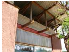
SCREWS POSITION SCREWS MUST BE PLACED IN THE CROWN OF RIDGES
