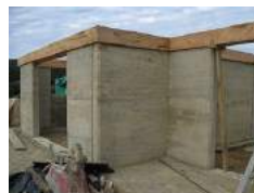
CONCRETE BEAM TO REINFORCE RAMMED WALLS
