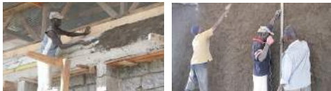
EARTH BAG WALL BEING COVERED BY CLAY COATING
