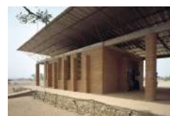
METAL FRAMED ROOF WITH LOADBEARING BRICK WALL SYSTEM. BRICK PILLARS HELP CARRY THE LOAD OF THE ROOF.
