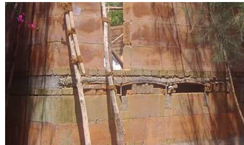
STONE FOUNDATION WITH MUD BRICKS, RAMMED EARTH WALLS CAN HOLD WELL IN PLACE ON ITS OWN WEIGHT, THE MUD BRICKS ARE THERE FOR DECORATION AND ARE OPTIONAL.
