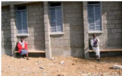
WINDOWS WITH VERTICAL SHADING DEVICES (PROTRUDING STONE UNITS), SHUTTERS, AND AN UPPER WINDOW FOR VENTILATION
