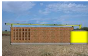
BOTTOM: THE CISTERN, CONNECTED TO THE SLOPED ROOF FOR STORING RAINWATER THROUGHOUT THE YEAR.
