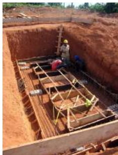
COMMUNITY MEMBERS HELPING WITH SITE EXCAVATION AND THE FORM WORK FOR THE FOUNDATION.
