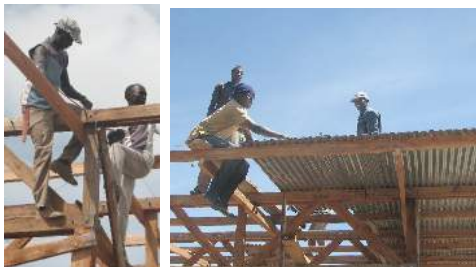
THE ROOF CONSISTS OF CORRUGATED METAL AND IS RAISED FROM THE INTERIOR ROOF BY WOODEN TRUSSES CONSTRUCTED ON THE GROUND AND THEN FASTENED IN PLACE. THE TRUSSES ARE LINED WITH TRADITIONAL SHANGA FABRIC MADE BY LOCAL WOMEN.
